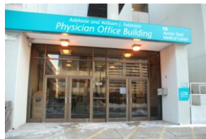
From Kilbourn Ave (1 st floor, South)
